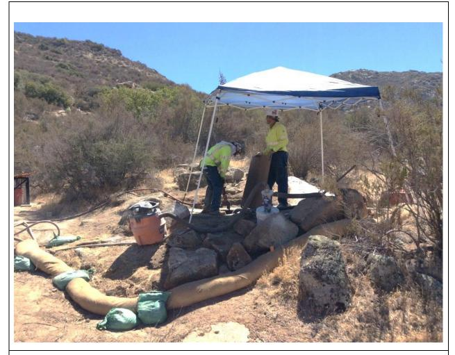
**Photo 3:** The hand digging crew at Pole P258090 (C 157) was observed using a containment system to capture dust emissions from rock jackhammering, in accordance with APM AIR-05.
