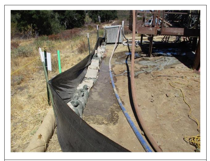
**Photo 5:** During micropile drilling at Z40517 (TL 629C), silt fencing and a gravel bag berm were installed along the downslope side of the work area to contain groundwater from being expelled from the drill hole, in accordance with the Erosion Control Plan and SWPPP.
