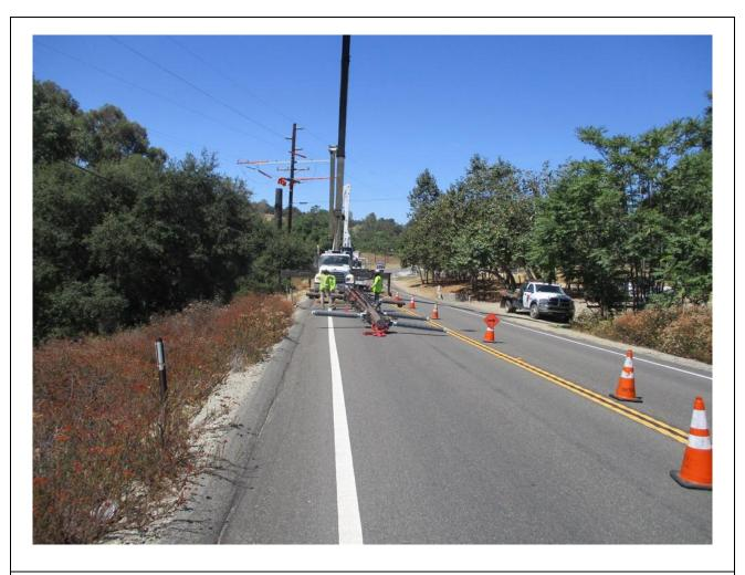
**Photo 6:** During pole framing and installation at Z112236, crews implemented a lane closure along Highway 76 in accordance with APM TRANS-02.
