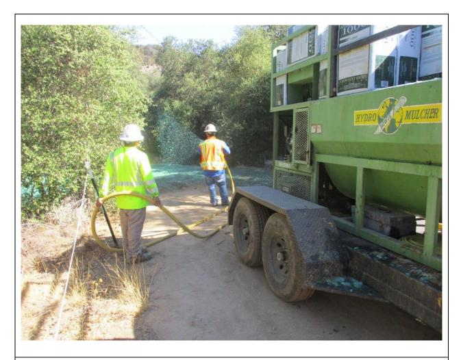
**Photo 2:** A crew is observed applying hydromulch at Z118153 (TL 682), in accordance with the Erosion Control Plan and SWPPP.
